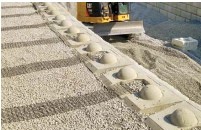
Figure 21 – Remove Slack in Top Side of Grid
