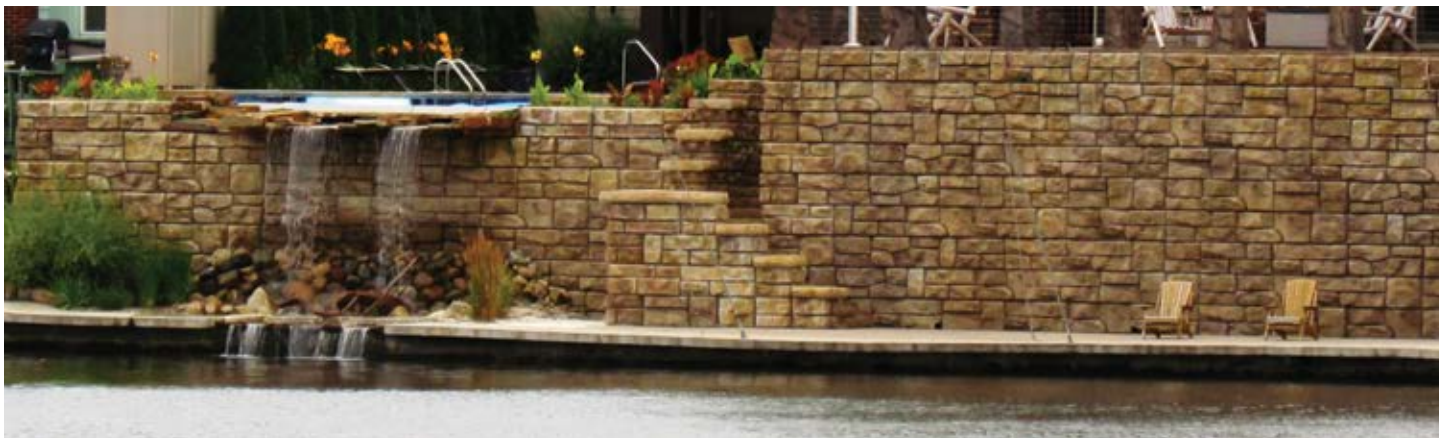
Figure 34 - Water feature part of Redi-Rock wall
