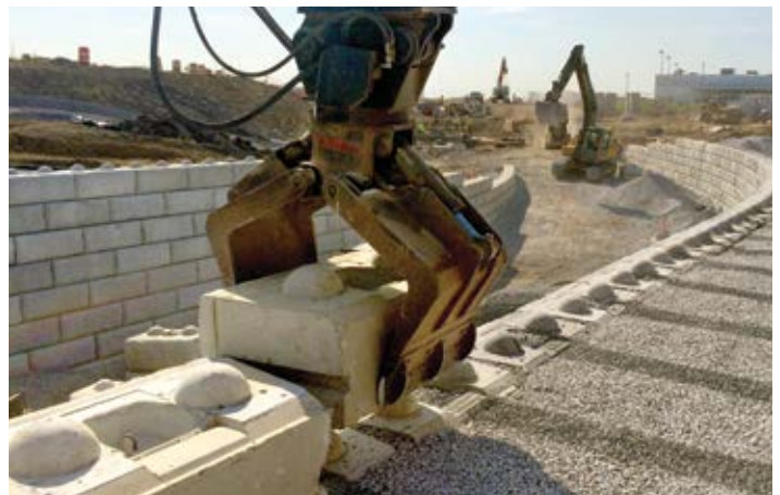
Figure 22 – Continue Block Placement
