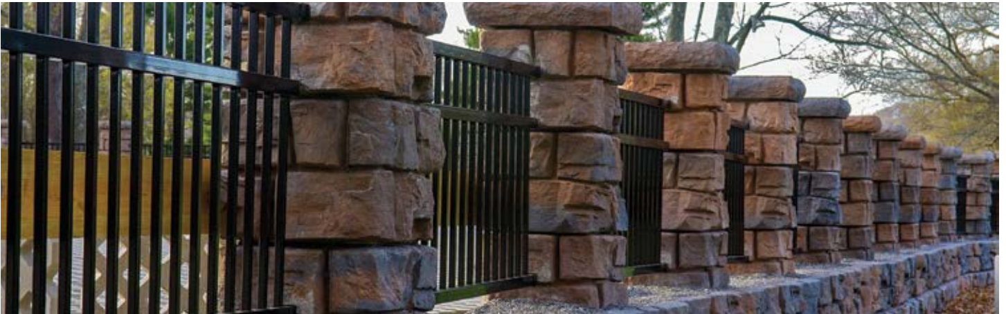
Figure 33 – Finished Redi-Rock Columns
