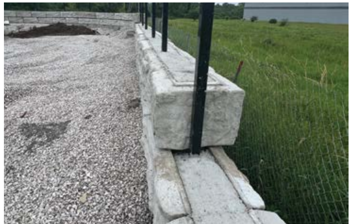
Figure 29 – Completed Hollow-Core Block Coping
