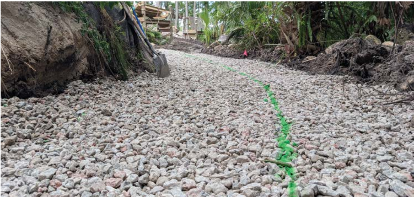
Figure 6 – Spray Paint can be Used for Staking
