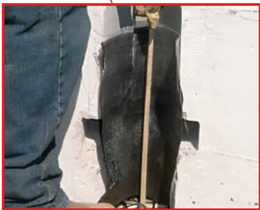
Figure 11 – Placing Non-Woven Geotextile Fabric
