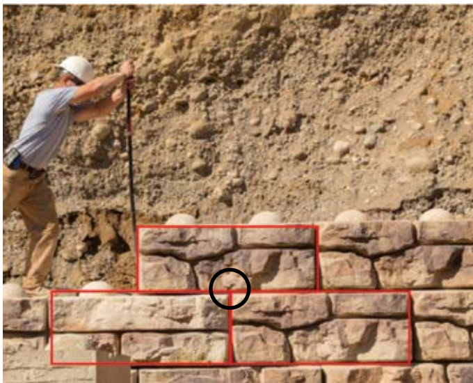
Figure 15 – Running Bond Configuration
