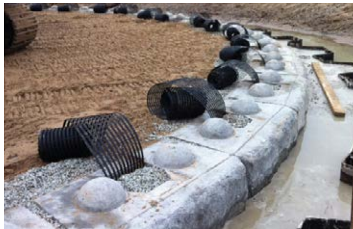
Figure 20 – Installed Drainage Aggregate
