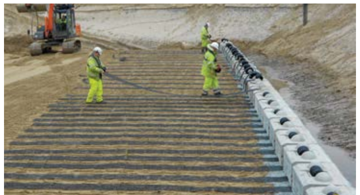
Figure 18 – Remove Slack in Bottom Side of Grid
