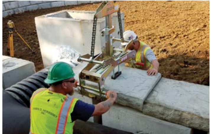
Figure 31 – Installing Cap Using Clamp
