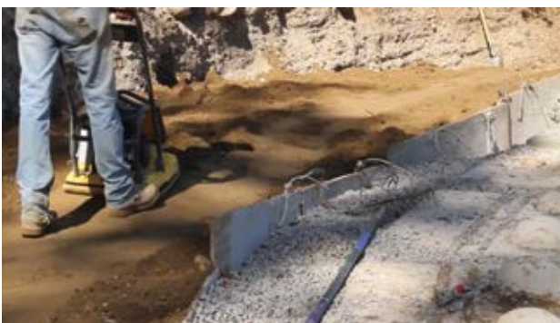
Figure 12 - Walk-Behind, Vibrating Plate Compactor
