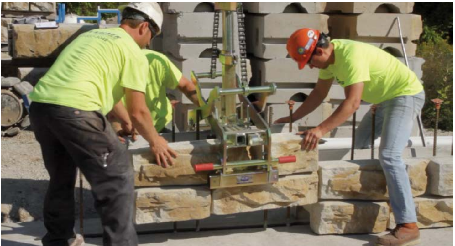
Figure 26 - Scissor Clamp for Block Placement
