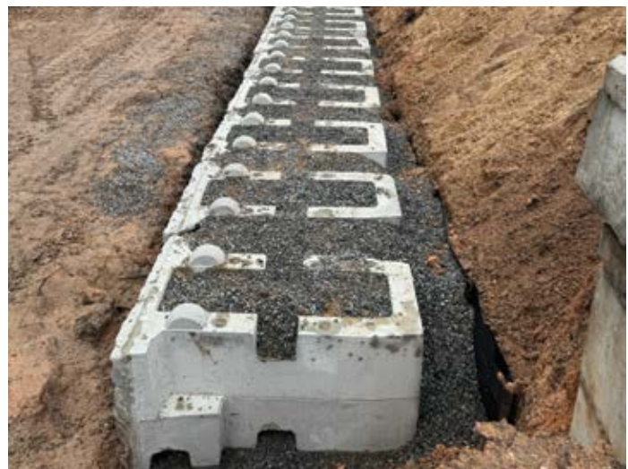
Figure 23 - XL Block with Stone Infill
