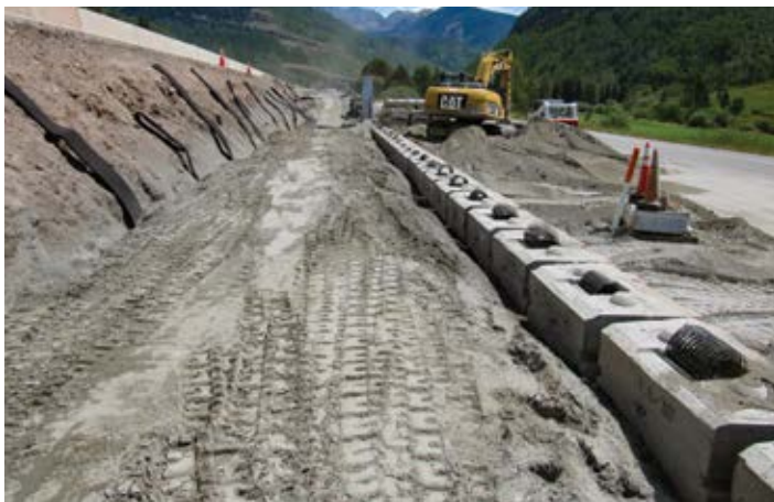
Figure 19 – Drainage Aggregate Locations
