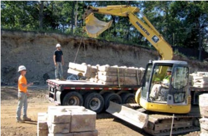
Figure 7 – Block Delivery on Site
