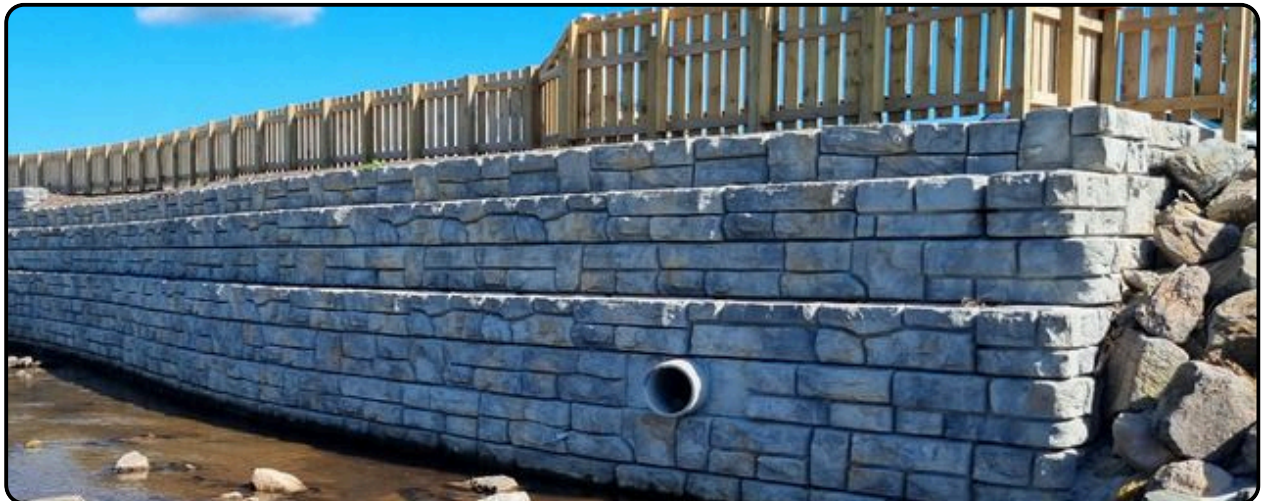
Figure 31 – Pipe Penetration Shown Through Wall
