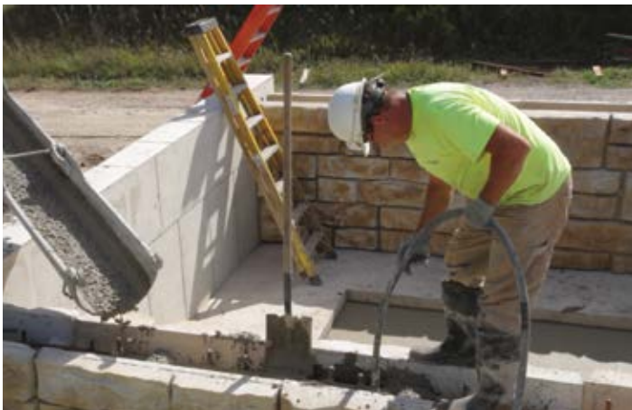
Figure 28 – Fill Hollow Core with Cast-In-Place Concrete
