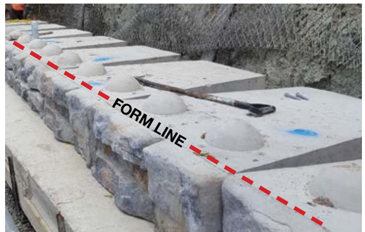
Figure 10 - Form Line Alignment
