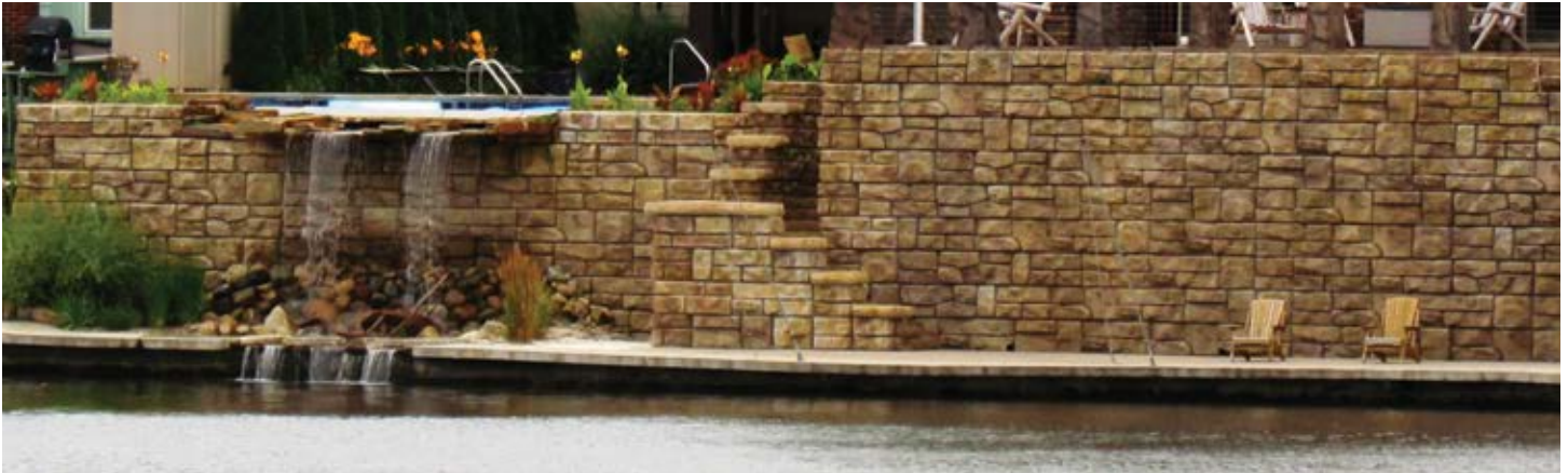
Figure 34 - Water feature part of Redi-Rock wall
