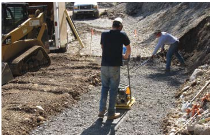
Figure 3 – Walk-Behind Plate Compactor on Subgrade Soils
