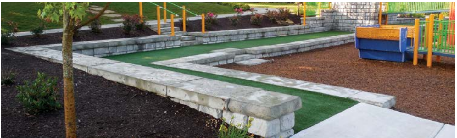
Figure 35 - Turf area in between tiered walls
