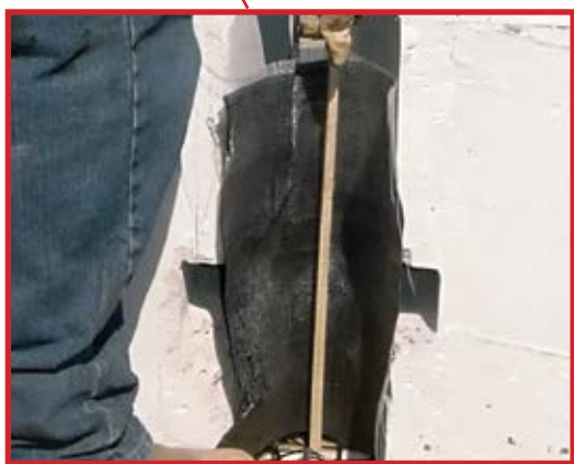
Figure 11 – Placing Non-Woven Geotextile Fabric
