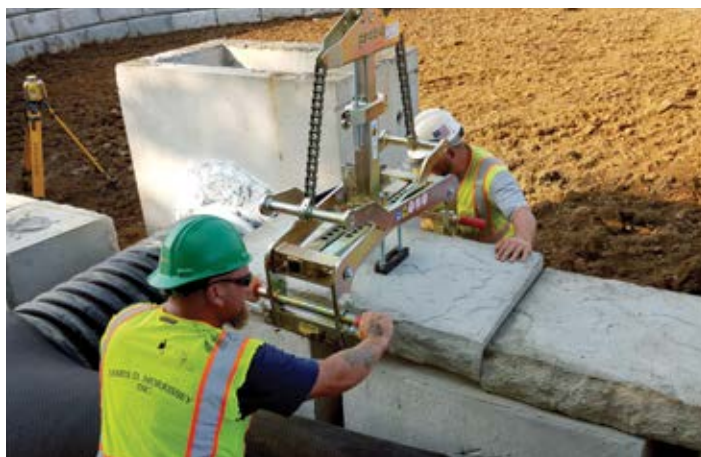
Figure 31 – Installing Cap Using Clamp
