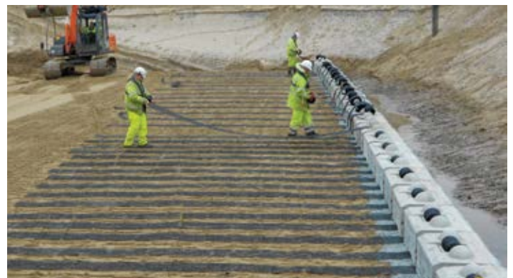
Figure 18 – Remove Slack in Bottom Side of Grid
