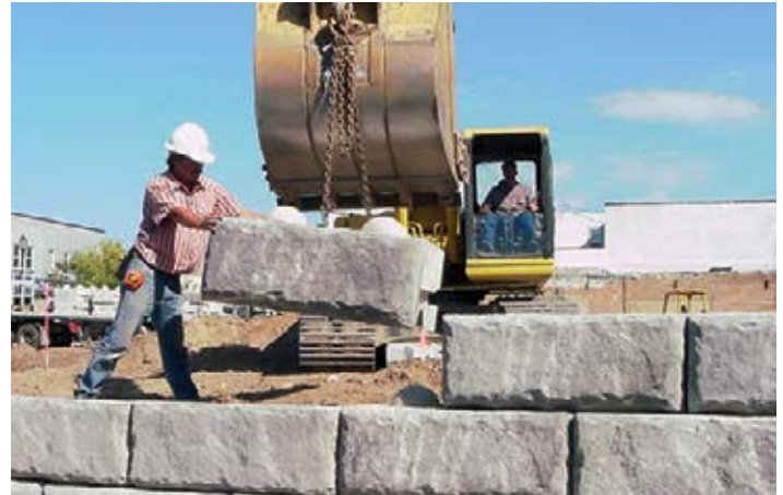
Figure 8 – Excavator Placing a Block
