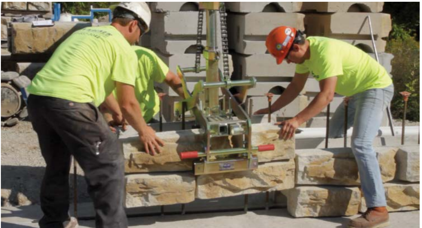
Figure 26 - Scissor Clamp for Block Placement
