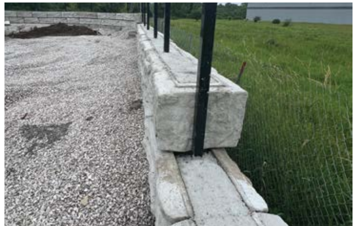
Figure 29 – Completed Hollow-Core Block Coping
