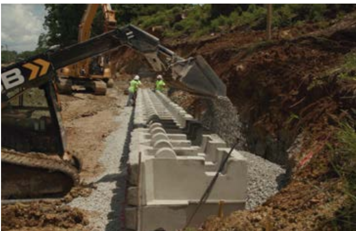
Figure 13 – Backfill Material
