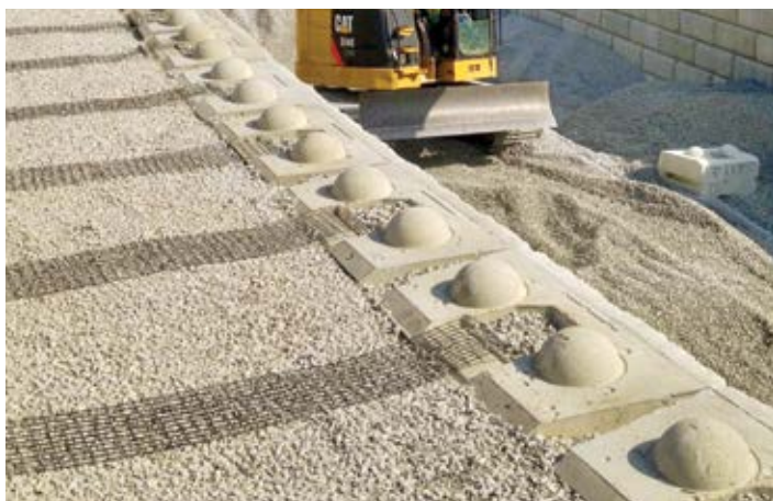
Figure 21 – Remove Slack in Top Side of Grid
