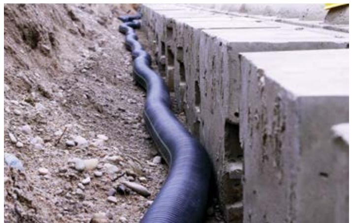
Figure 14 - Placing the Wall Drain
