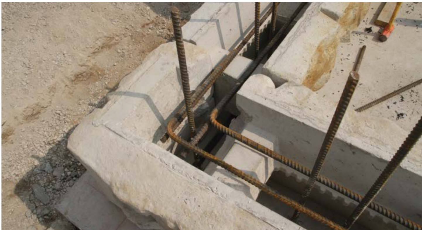
Figure 27 – Rebar in Grooves Ready for Concrete Fill
