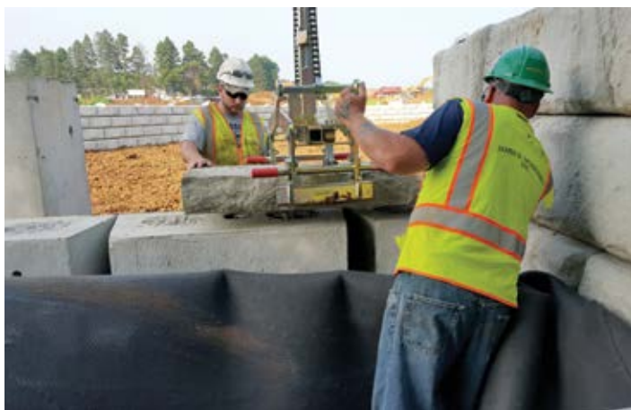
Figure 30 – Installing Cap on Retaining Block
